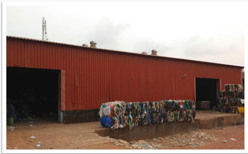
Verna MRF (outside view)
